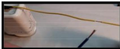
4. Lay the stripped end of the wire to be joined over the bare section of the existing wire.
