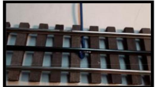
12. Drill about a 1/8 inch to 3/16 inch hole through the layout next to the solder joint.
