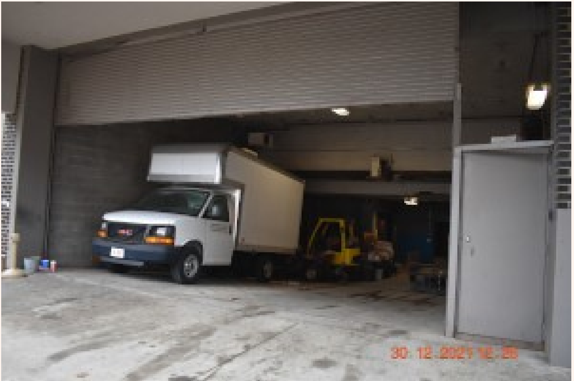
Loading Dock with one door open. Freight elevator to left of the fork lift
