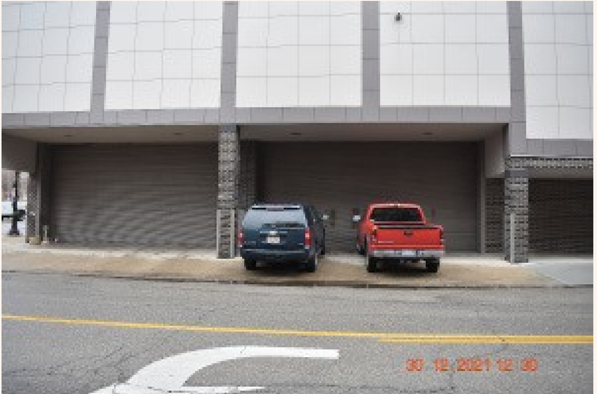
Loading Dock Doors on Market Street
