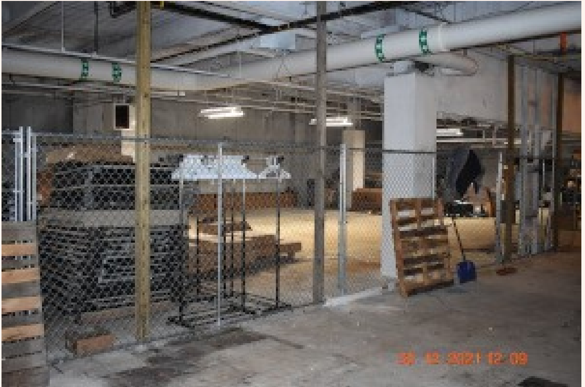
Star Tec Fenced in area Wood uprights for fence support.
